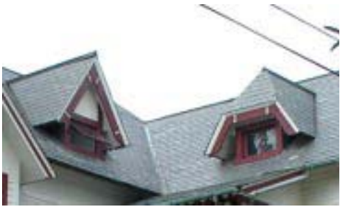
Detail of Pearce House showing slate roofing
