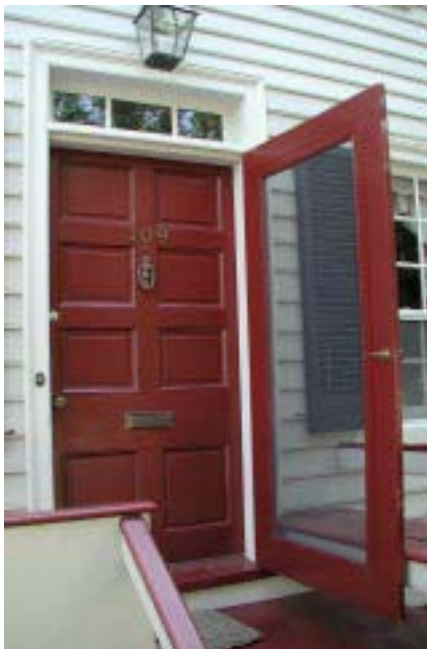
Doorway with appropriate storm door
