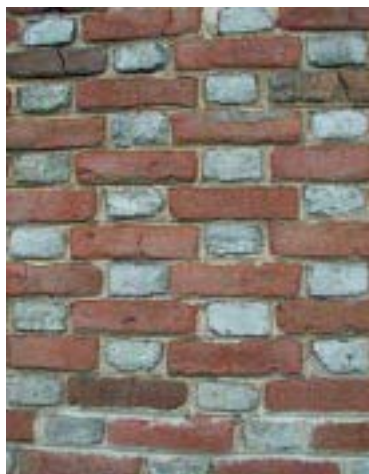
Flemish Bond with glazed header bricks
