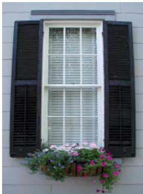
Sash window with louvered shutters
