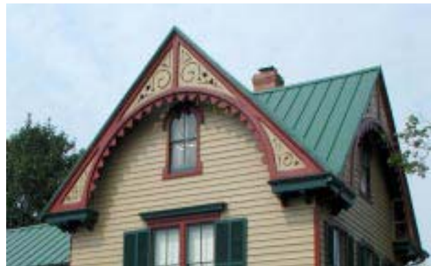
Detail of Boyd House showing metal standing seam roof
