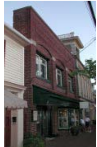
Parapet wall, Cross Street
