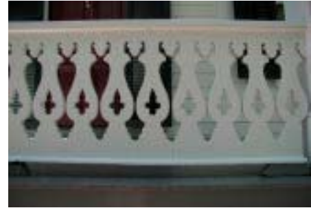
Wood porch railing, High Street
