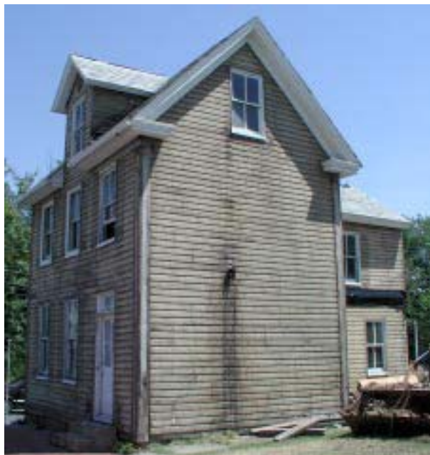
House on Mill Street being prepared for moving
